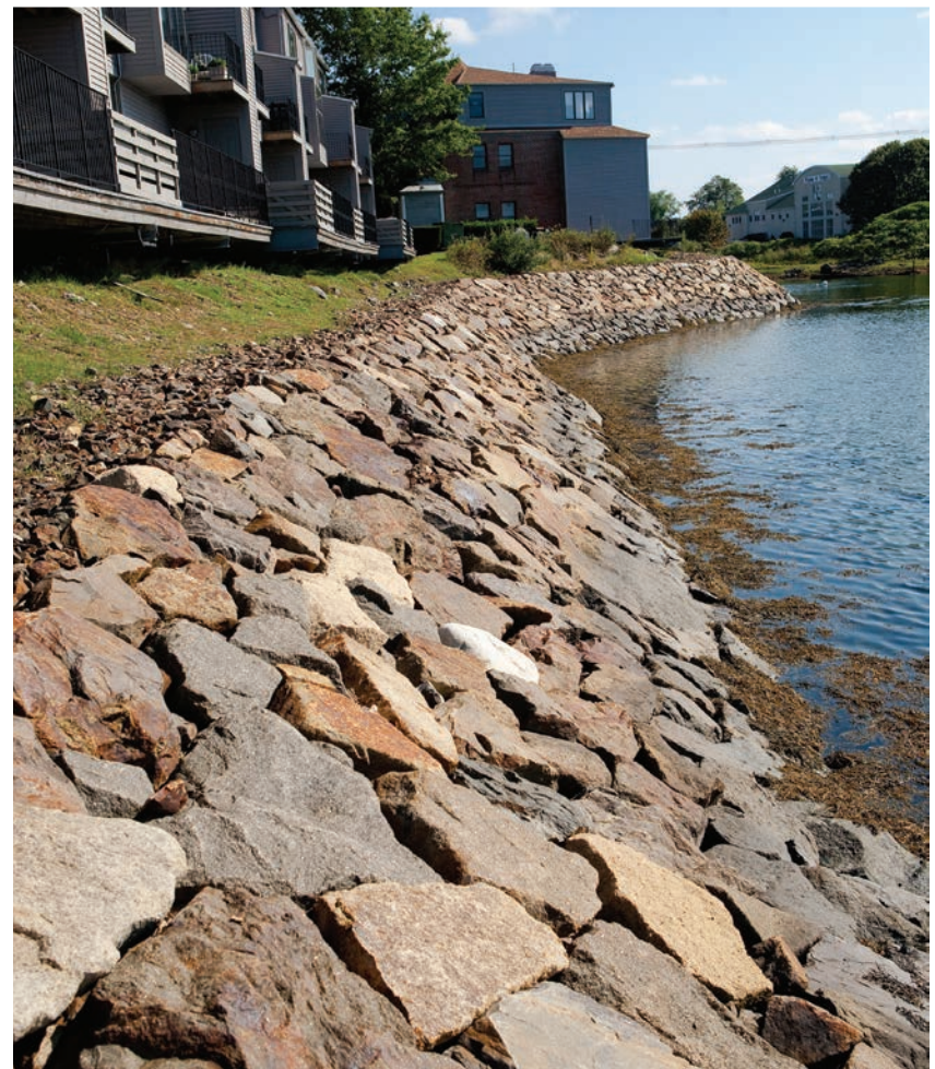
Rip Rap shoreline stabilization project. Nobles Island, Portsmouth, NH
