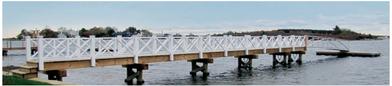
3.5' x 35' custom arched aluminum gangway with red cedar decking and handrails. Cape Porpoise Harbor, ME
